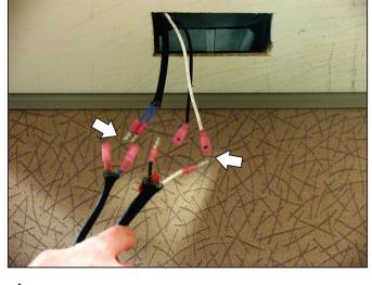
Pull the transformer wires out until the terminals are accessible.
